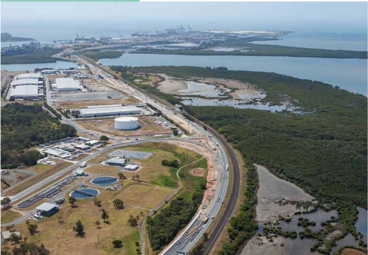
Port Drive upgrade under construction 2018
